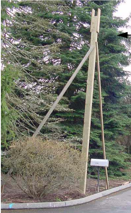
Overhead Temporary Clearance Pole
