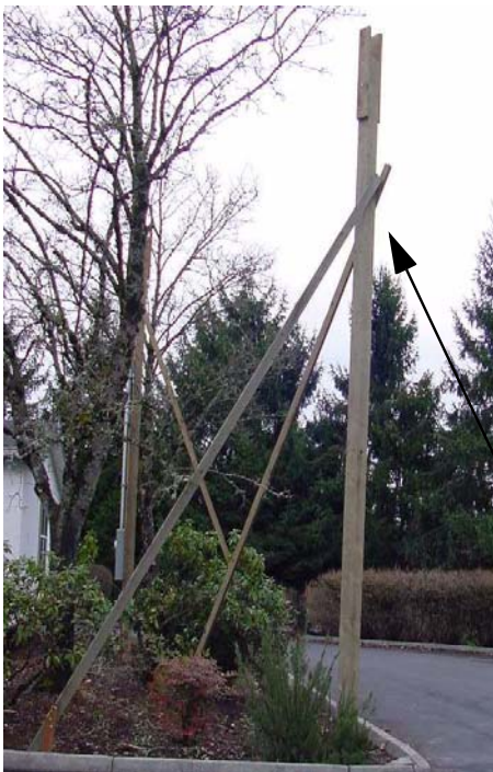
Overhead Temporary Clearance Pole
