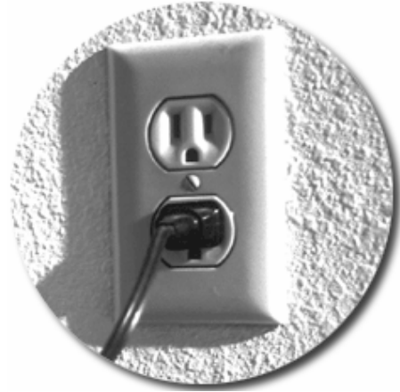
120 Volt Outlet: Supplies electricity to most home appliances.
