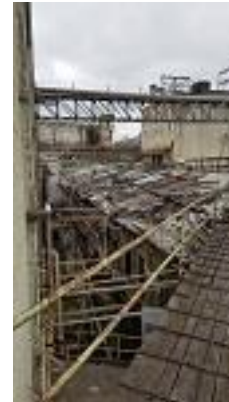
Mill J roof
